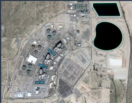
Palo Verde Plant, Arizona || 2019
